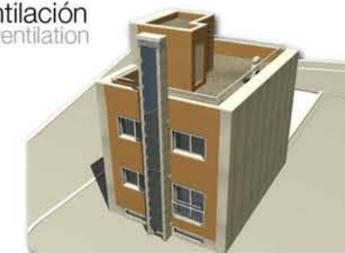
chimenea solar solar chimney
